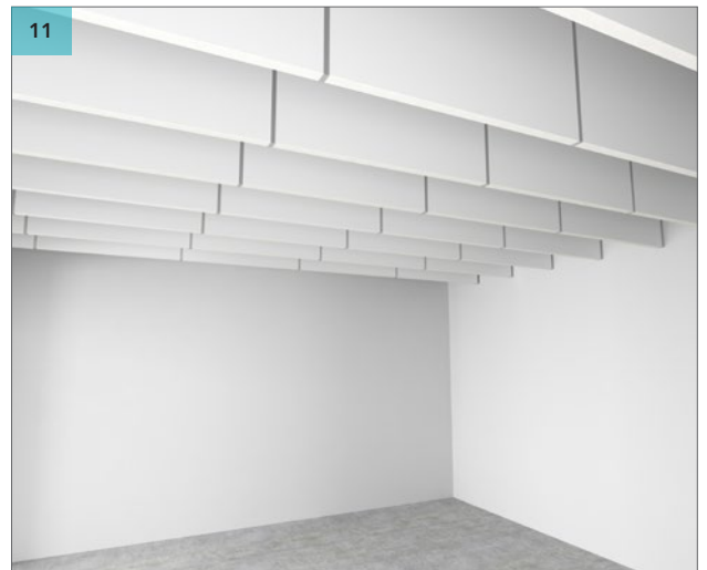
Fix all the remaining baffles in the room.
