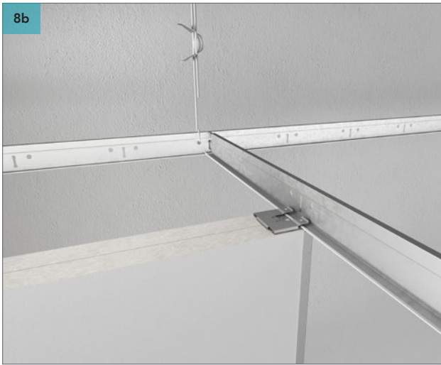
Fix baffles to the suspended T24 profiles. You can use the slots of the T24 profiles to align the baffles.
