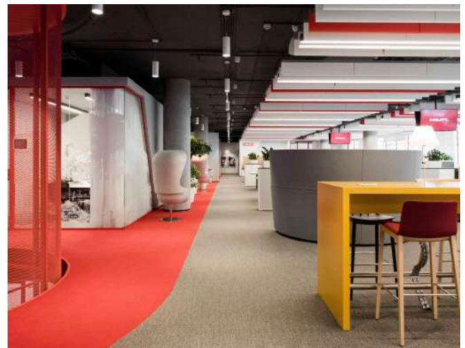
Baffles in a commercial setting
